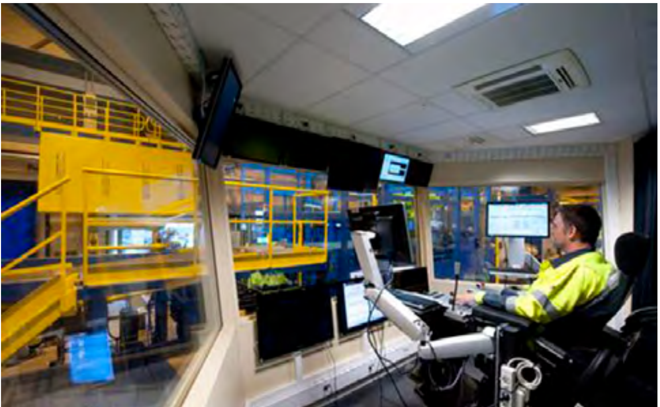
▲ Modern Main Control Desk of Heavy Gauge CTL lines
